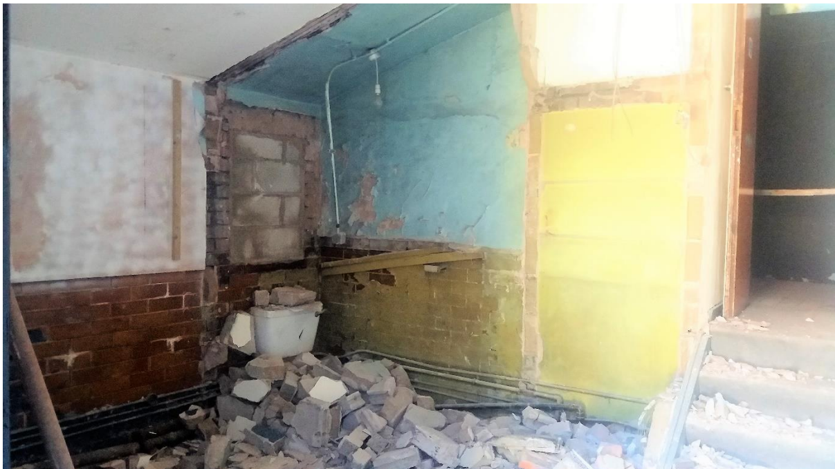
Above Like so many disused spaces 'the old kitchen' was actually storing junk. The black shape to the left was a nailed-up door. It is now a new, additional emergency exit. Below Gutting the room before creating the stud walls.
