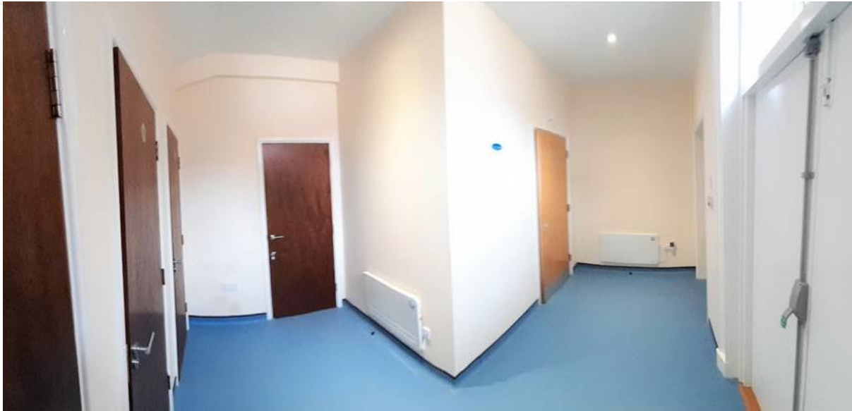
Panorama image of the new toilet block.
